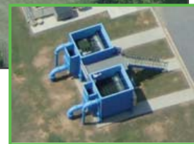
Aerial of the 2-basin AquaSBR ® system with adjacent (2) 6-disk AquaDisk ® filters.
