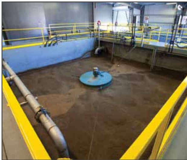
One of Quechan Casino's batch biological reactors.
